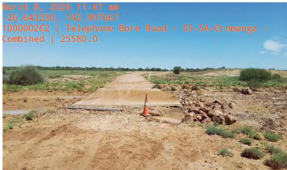
Photo above Telephone Bore Road Ch 25,590
