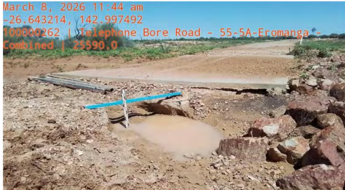
Photo above Telephone Bore Road Ch 25,590
