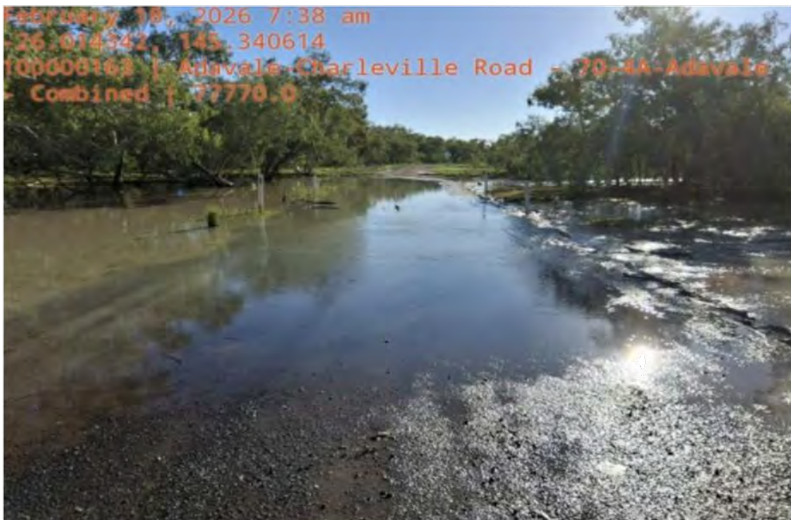
Photo above of Ambathalla Lakes Crossing.
