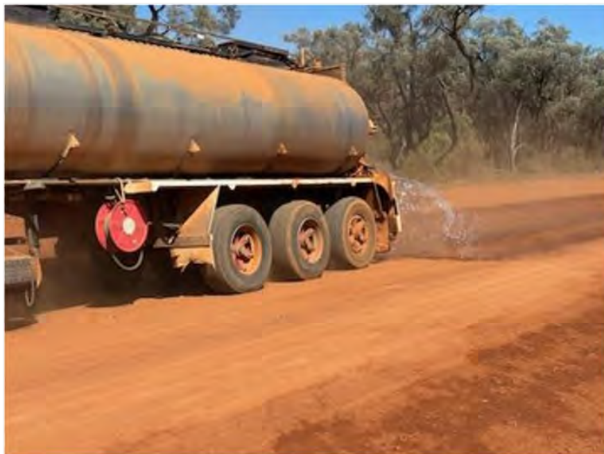
Photo above shows constant addition of water during the construction phase.
