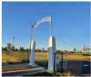
1 ENTRY GATE ON CHIPU STREET IN DISREPAIR - NEW PAINT REQUIRED
