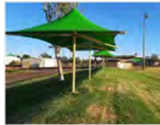
3 SPECTATOR MOUNDING POSES A DISCONNECT BETWEEN CHANGE ROOMS AND FIELD - POTENTIALLY CUT GAP OR TUNNEL AND EXTENT MOUNDING TO THE SOUTH
