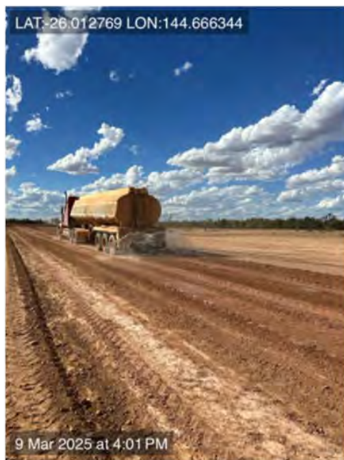
Application of water during REPA construction works on Cheepie Adavale Road.
