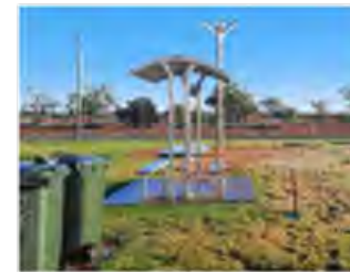
19 SMALL PICNIC SHELTER DOES NOT PROVIDE ADEQUATE SHADE DUE TO SMALL ROOF SIZE – TO BE REMOVED
