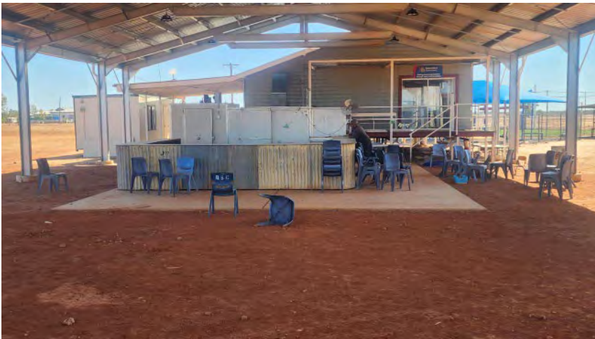
Figure 1 Adavale Sport and Recreation Grounds shed
