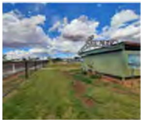
GATES FACING ROAD ARE NOT SELF-CLOSING AND POTENTIAL RISK OF CHILDREN ENTERING ROAD - IMPLEMENT SELF-CLOSING AND LOCKING GATES
