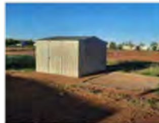
8 SMALL STORAGE SHED AND CONCRETE SLAB SERVE NO PURPOSE - REMOVE
