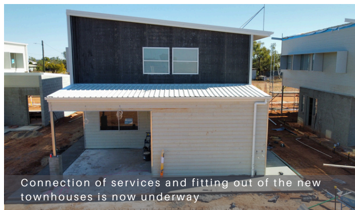
Construction of the new townhouses
