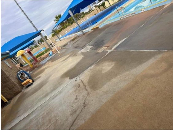
Pool deck post pressure cleaning
