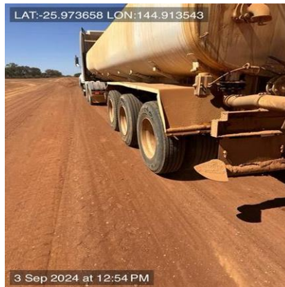
Proof rolling by Proterra Group staff of work completed.
