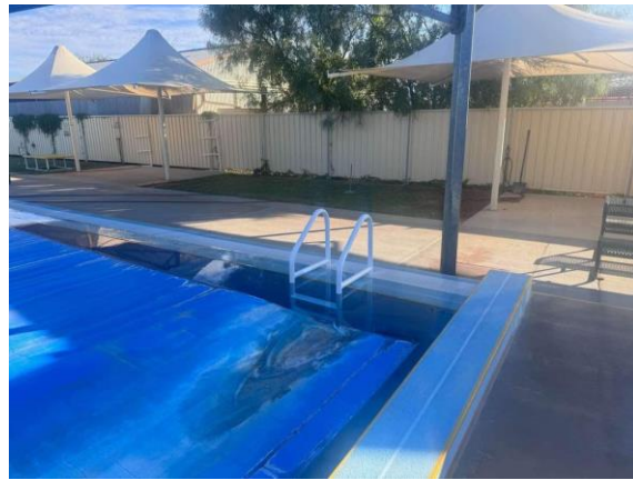
Ladders installed 25 metre pool
