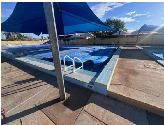
Depth indicators installed
