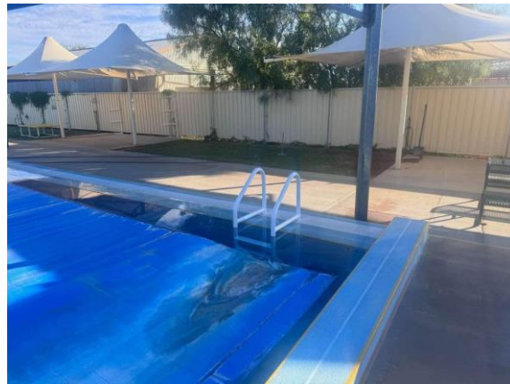
Ladders installed 25 metre pool
