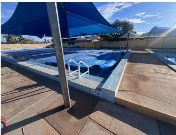
Depth indicators installed
