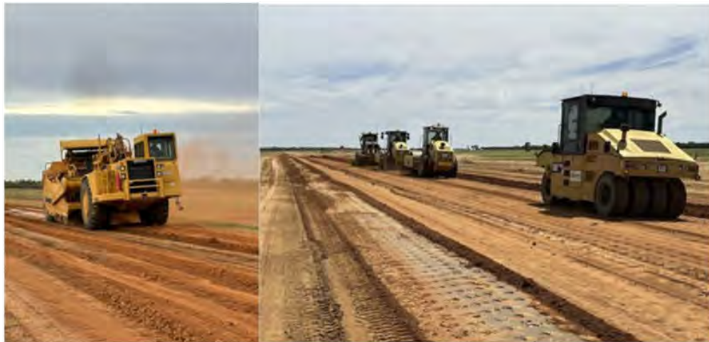
Machines busy on Adavale Black Road
