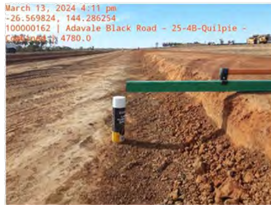
Replacement of Sub Base layer on Adavale Black Road
