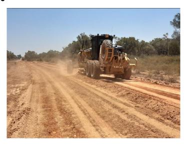
Grader used for profiling of existing material plus inclusion of new material where specified.
