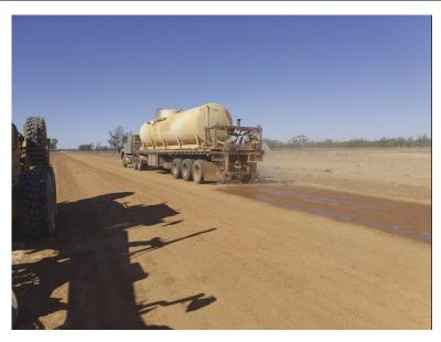
Water Tanker used to cart water for construction of roads, plus backwatering where required.
