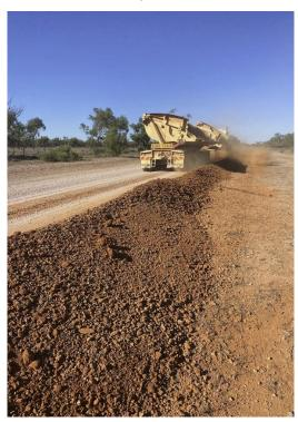
Material which has been prepared in registered pits are hauled to site and rilled along the road. This material will be used to replace material which has been lost.
