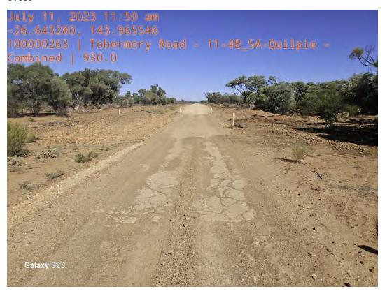
This section was previously protected by a concrete floodway. However, this concrete has reached its end-of-life span and has disintegrated, and due to this is now becoming a hazard to light vehicles. There is no under road drainage. Recommendation is to reconstruct concrete floodway between new upper and lower concrete margins.
