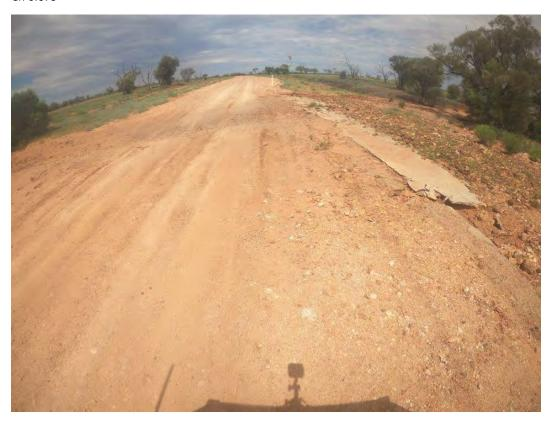
Though there is currently no protection in place, this same area gets damaged many times a year and the damage is severe enough after minimal rainfall that it leads to damage to vehicles.
