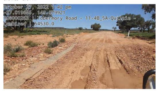
The above floodway was constructed too short and the section that is not concrete gets damaged regularly, being very close to the homestead this damage triggers complaints often. The recommendation is to extend the existing floodway a further 20m between the two concrete margins.
