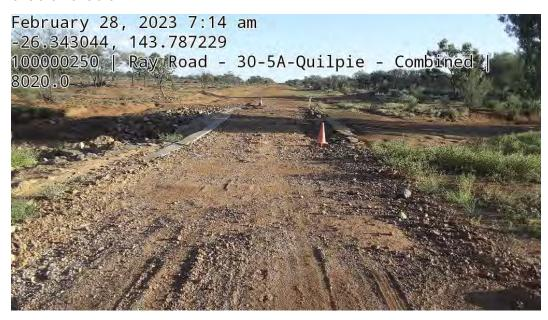
This area has previously been stabilized, however due to the nature of the overland flow in this area, this site gets repeatedly damaged. Recommendation is to construct concrete floodway between upper and lower concrete margins. There is currently under road drainage in place, however due to low lying nature of area this pipe is full of sediment and is expected to remain the same way.
