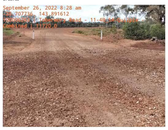
Though there is currently no protection in place, this same area gets damaged many times a year and the damage are severe enough after minimal rainfall that it leads to damage to vehicles.
