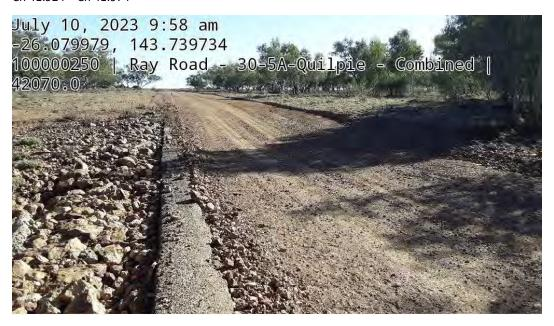
This area has previously been stabilized, however due to the nature of the overland flow this area gets repeatedly damaged. Recommendation is to construct concrete floodway between existing upper and lower concrete margins. There is currently no under road drainage in place, and none are planned. Overall length 50m by 6m wide
