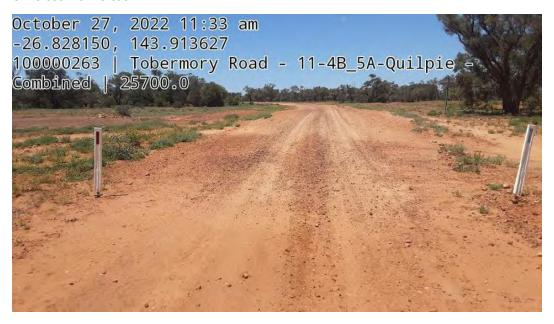
This section was previously protected by a concrete floodway. However, this concrete has reached its end-of-life span and has disintegrated, and due to this is now becoming a hazard to light vehicles. There is no under road drainage. Recommendation is to reconstruct concrete floodway between new upper and lower concrete margins.
