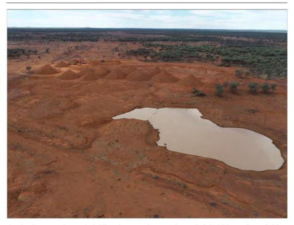
Contractor screening material thereby removing oversize material whilst ensuring suitable quality material is being prepared for inclusion into the REPA works near Toompine.
