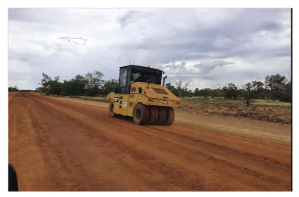
Part of the process is to compact the material which has been prepared using this Multi Tyre Roller, this will ensure longevity of pavement and maintain crossfall.
