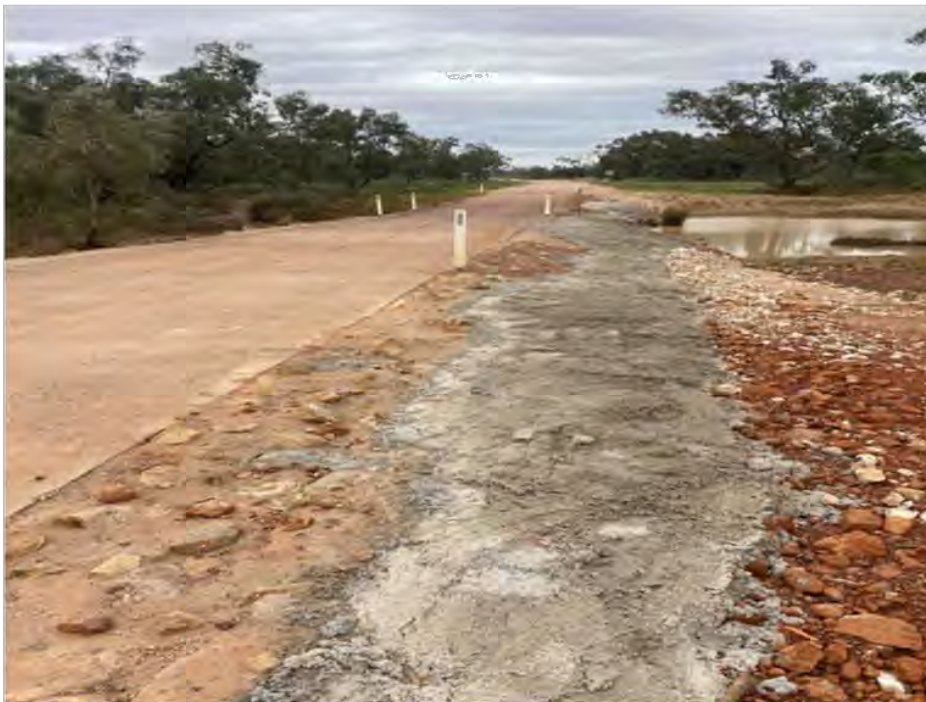
Minor flowable concrete works on Adavale Black Road
