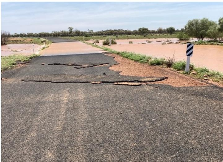
There is massive damage to some roads, where the pavement is saturated and full of water. Council is trying to keep traffic off these roads until the pavement can dry out enough to perform reconstruction works.
