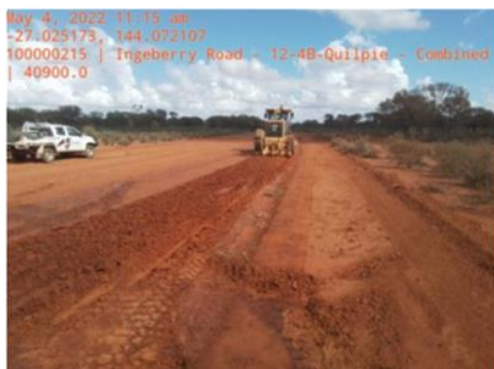
Ingeberry Road, preparation for Heavy Formation Grade
