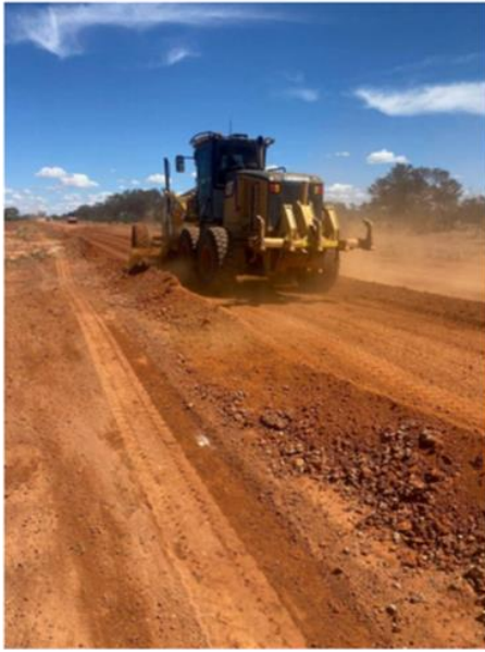
Preparation of material before inclusion into pavement.
