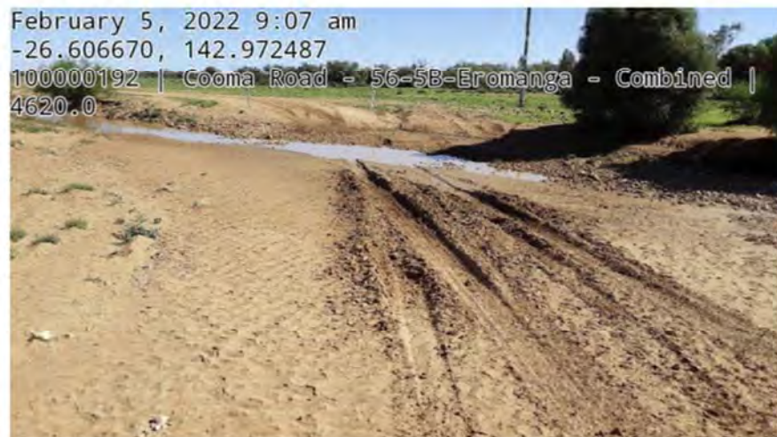
Emergent Works on Cooma Road-5 February 2022.
