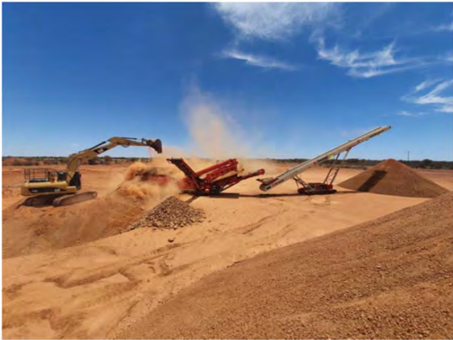
Preparation of material by screening contractor at the Congie Road pit.
