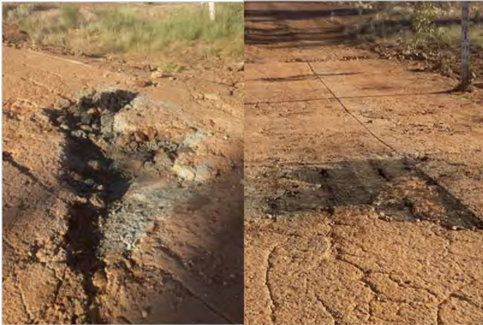
Concrete floodways that have reached end of life cannot be repaired under QRA funding.
