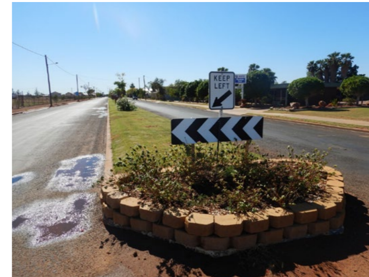
2.3. Brick retainer around end gardens of all median planters looks untidy
