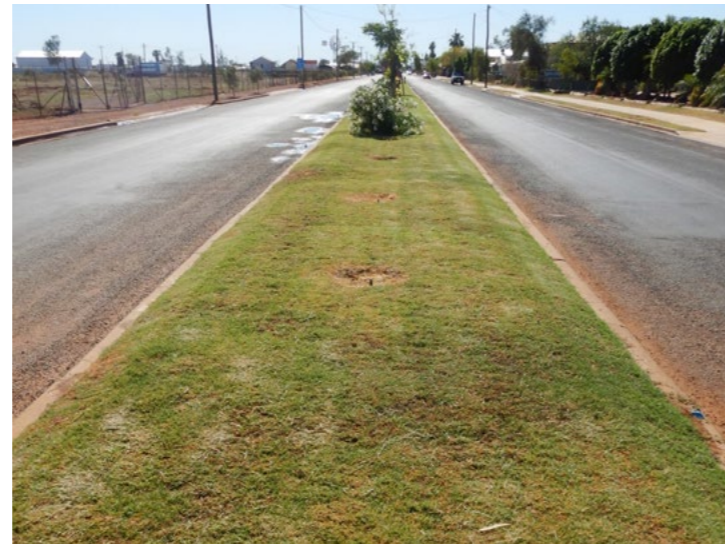
2.2. Irrigation running in centre of median and overspraying onto road
