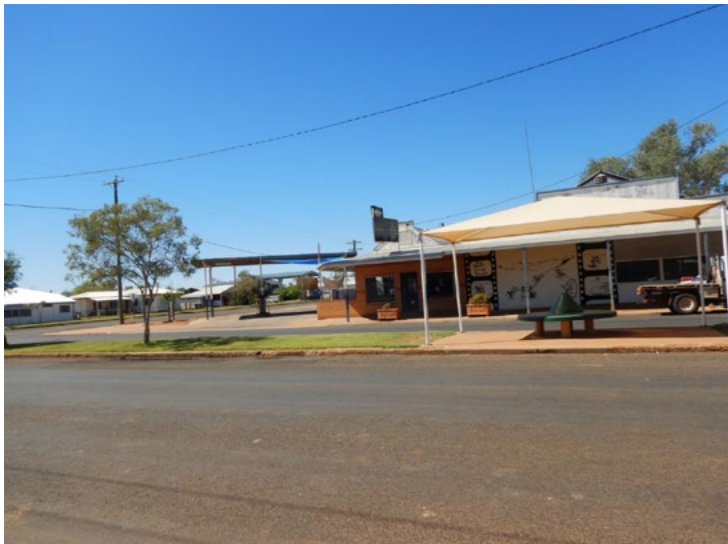
2.1. Shade structures with seating appear unsafe as people need to cross the road to use them
