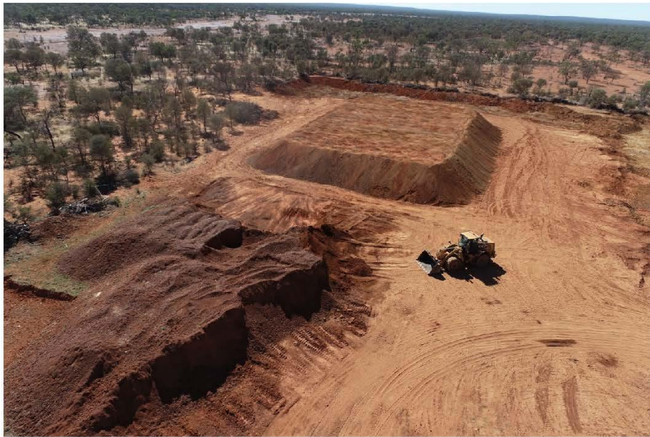
Screened material at Pit # 32-ready for inclusion into Onion Creek Road and others.
