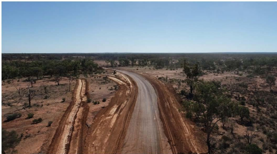
Initial works on Onion Creek Road clearing regrowth and degrading.
