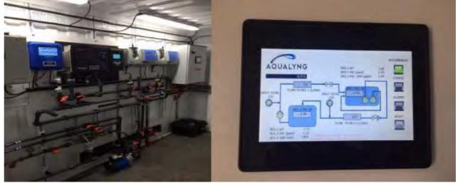
Analyser systems monitor free chlorine, temperature, conductivity, ORP, flow, circulation rates, product usages etc. Note control HMI is available as per HMI screen, online. All information communicated to WEB and securely accessible. To approved personnel.
