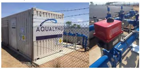
The system is installed in a fully power ventilated container, Chemical are separated and stored in a separate air extraction zone.
