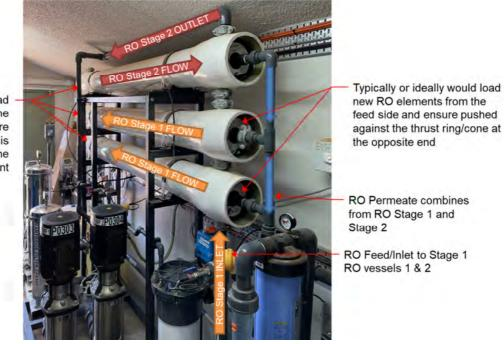
Should be possible to load new RO elements from the opposite end and ensure that thrust ring/cone is installed firm against the membrane element
