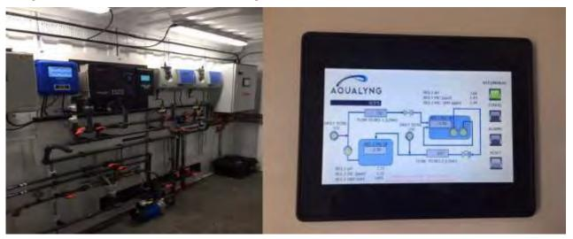
Analyser systems monitor free chlorine, temperature, conductivity, ORP, flow, circulation rates, product usages etc. Note control HMI is available as per HMI screen, online.
