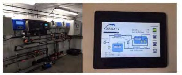
Analyser systems monitor free chlorine, temperature, conductivity, ORP, flow, circulation rates, product usages etc. Note control HMI is available as per HMI screen, online.
