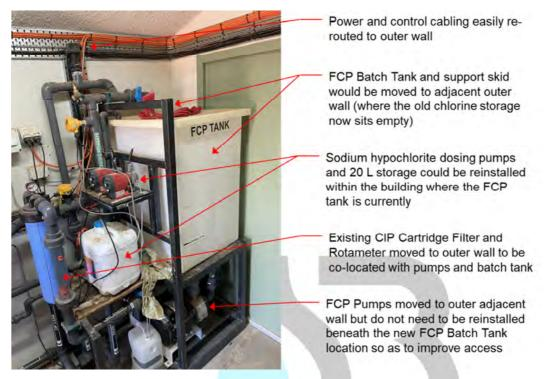
Figure 5: Installation details/requirements for moving CIP Tank and pump set
