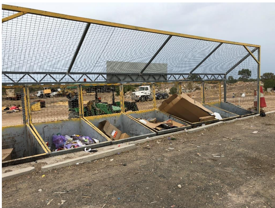
Figure 3-5 Transfer station proposed for QWMF comprised of front lift skip bins and litter fencing
