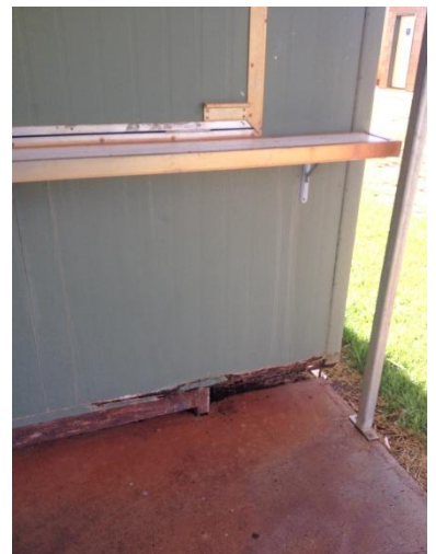
Rust to substructure Bar building
