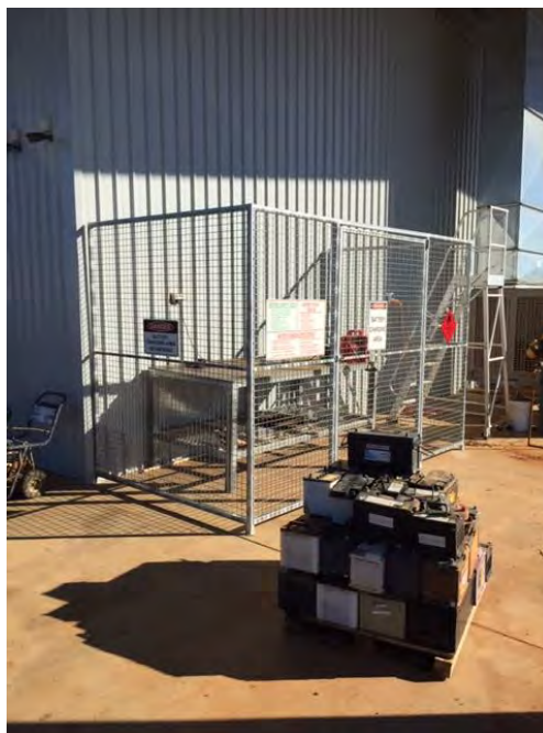
Battery charging station cage installed
