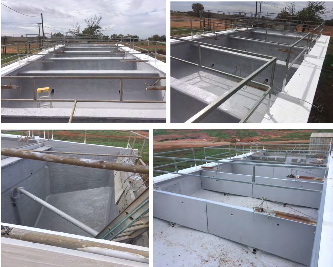
Sewerage Settling Tanks refurbishment & Baffles replaced
