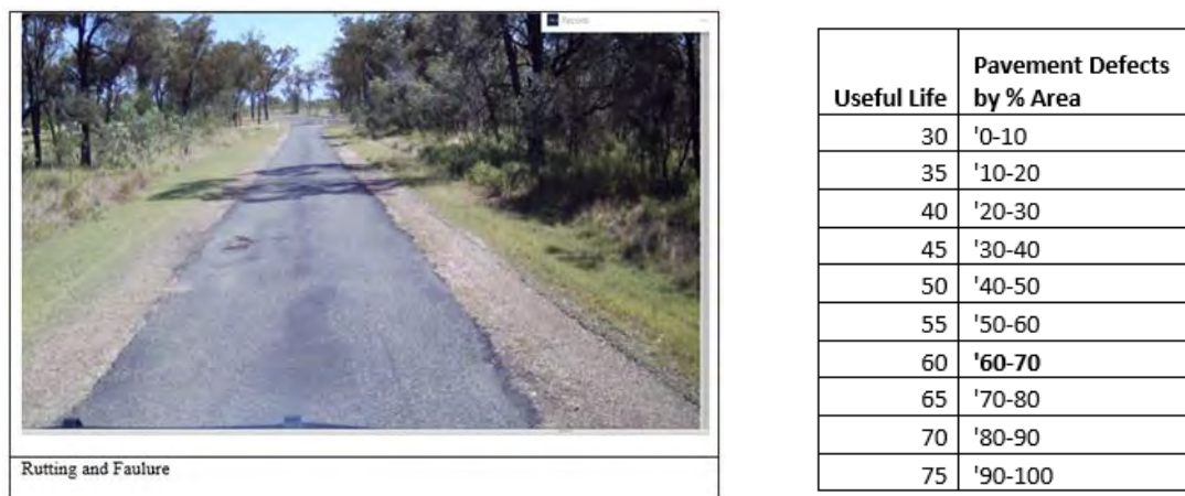
Figure 2.5.2.a Sealed Pavement Useful Life Relationship with % Area of Rutting and Failure Examples
