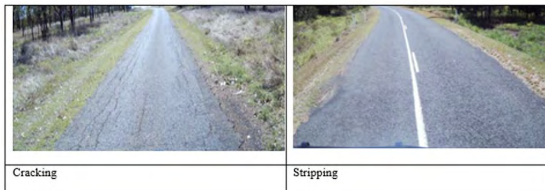
Figure 2.5.1.a Sealed Surface Cracking and Stripping Examples
